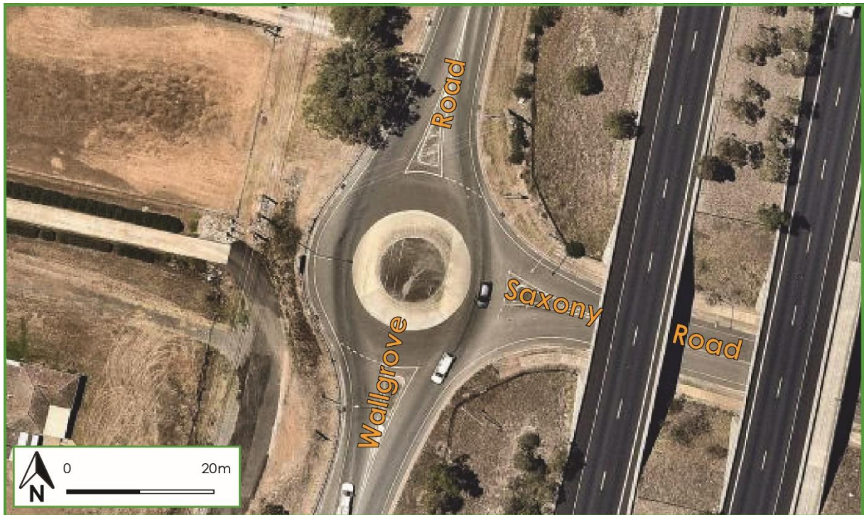
Figure 4: Intersection of Wallgrove Road with Saxony Road
